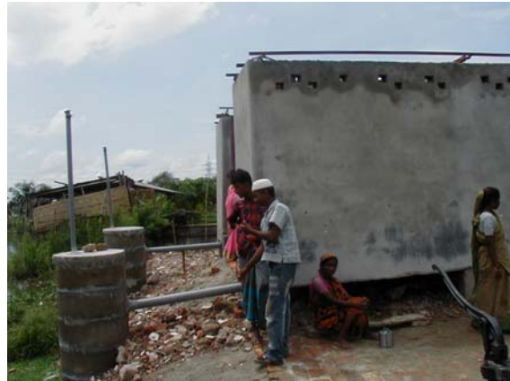
↑ A public toilet, now under construction in Dhaka City
