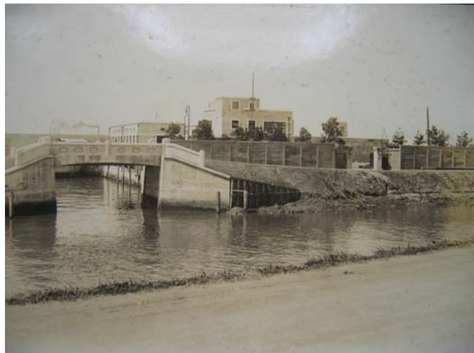
↑ Ayase night soil treatment facility
